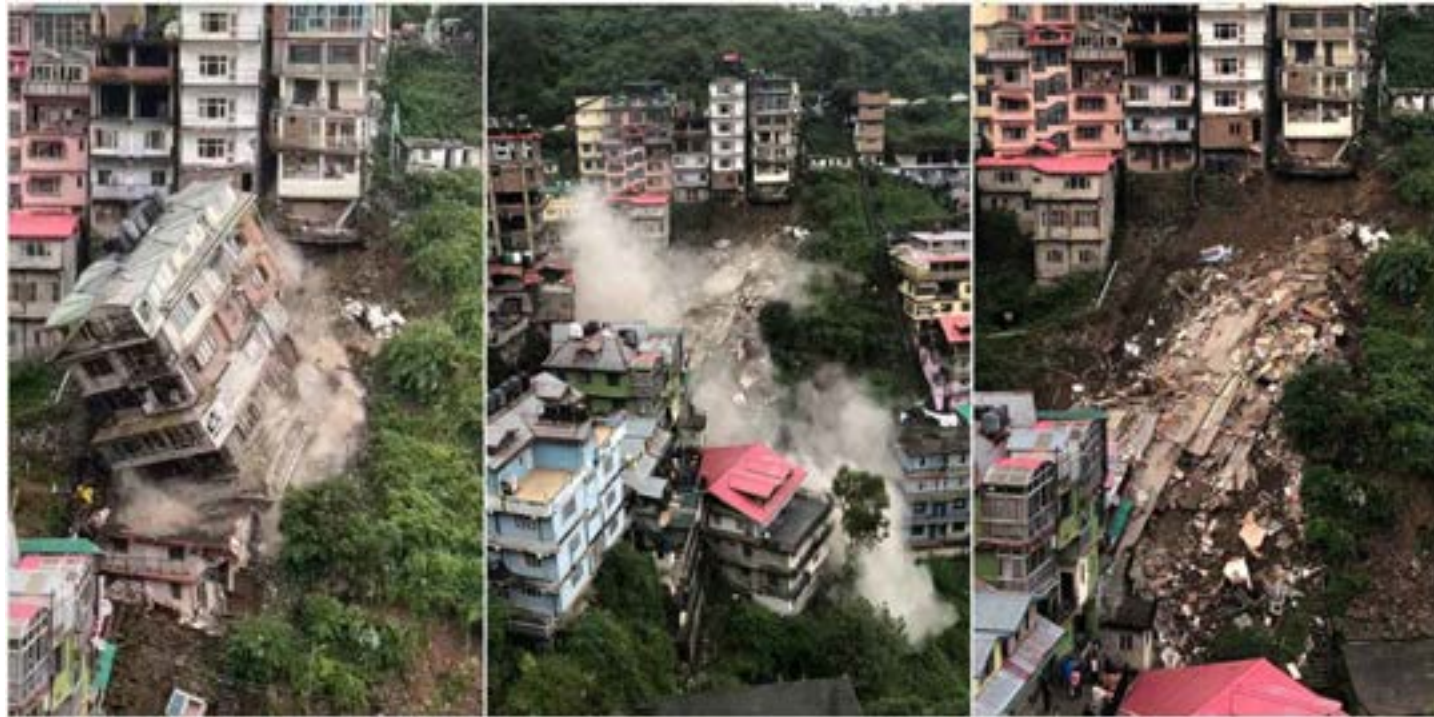
Image 4: The Collapse of an eight-story building in Shimla, 30 September 2021. Video by Amit Kanwar. For the full video go to: < https://www.tribuneindia.com/news/himachal/multi-storey-building-collapses-in-shimla-no-loss-of-life-318316 >. Bhanu Lohumi, 'Multi-Storey Building Collapses in Shimla,' Tribune News Service (Chandigarh, Haryana) 30 September 2021
