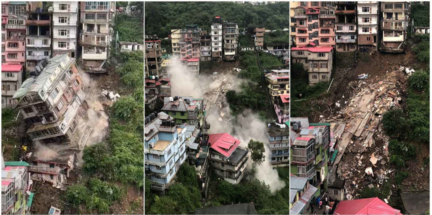
Image 4: The Collapse of an eight-story building in Shimla, 30 September 2021. Video by Amit Kanwar. For the full video go to: < https://www.tribuneindia.com/news/himachal/multi-storey-building-collapses-in-shimla-no-loss-of-life-318316 >. Bhanu Lohumi, 'Multi-Storey Building Collapses in Shimla,' Tribune News Service (Chandigarh, Haryana) 30 September 2021
